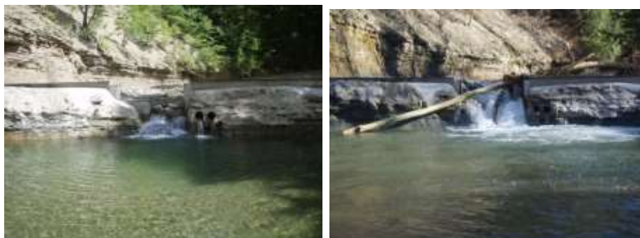
Figure 2d-2. Notching in the lower dam post-construction and pre-flood, and logs and rocks in notch after the Superstorm Sandy flood.
