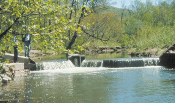
Low-head sea lamprey barriers prevent sea lampreys from reaching their spawning grounds. Once an effective sea lamprey barrier is constructed in a river, lampricide treatments are normally unnecessary above the barrier. Low-head barriers are usually equipped with devices to pass fish. PHOTOS: GLFC, A. HALLETT
