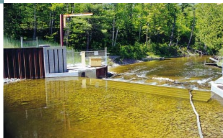
Low-head sea lamprey barriers prevent sea lampreys from reaching their spawning grounds. Once an effective sea lamprey barrier is constructed in a river, lampricide treatments are normally unnecessary above the barrier. Low-head barriers are usually equipped with devices to pass fish. PHOTOS: GLFC, A. HALLETT
